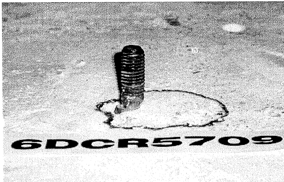
Figure 4.39 Yielding of Back Anchor and Spalling of Concrete for Double-Anchor Connection under Dynamic Shear Loading
